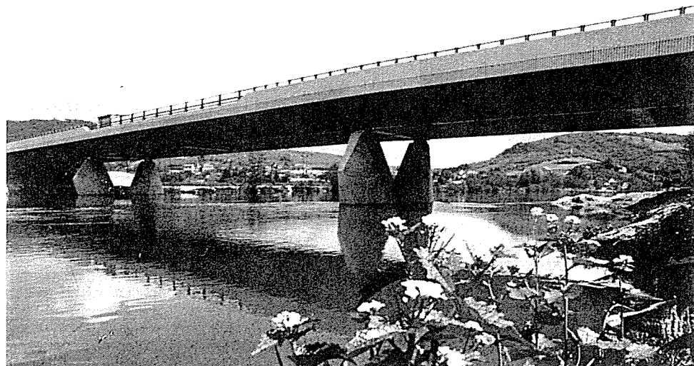
Workability and durability were two important HPC properties for Joigny Bridge.
